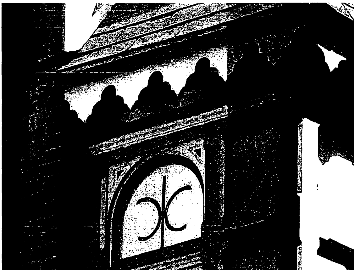
The Warner House also has an unusual second-story projecting bay paneled and decorated in wood. Left: The bay is supported by pairs of carved-wood brackets detailed with curvilinear "jig-saw" ornament. Top: The bay is also ornamented with wood panels and a bargeboard detailed with scalloped edging.
