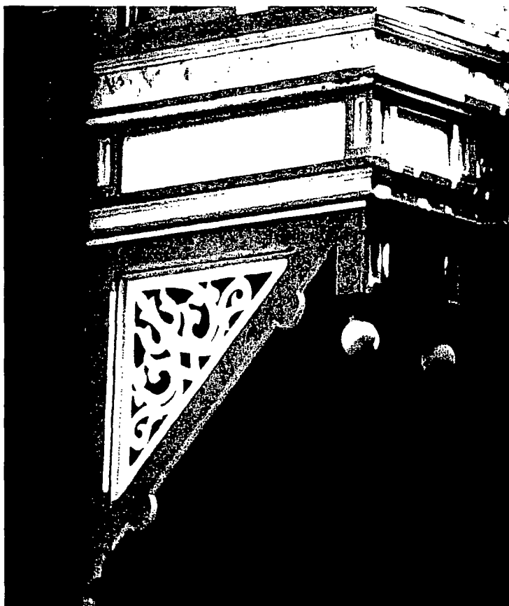
The Warner House also has an unusual second-story projecting bay paneled and decorated in wood. Left: The bay is supported by pairs of carved-wood brackets detailed with curvilinear "jig-saw" ornament. Top: The bay is also ornamented with wood panels and a bargeboard detailed with scalloped edging.
